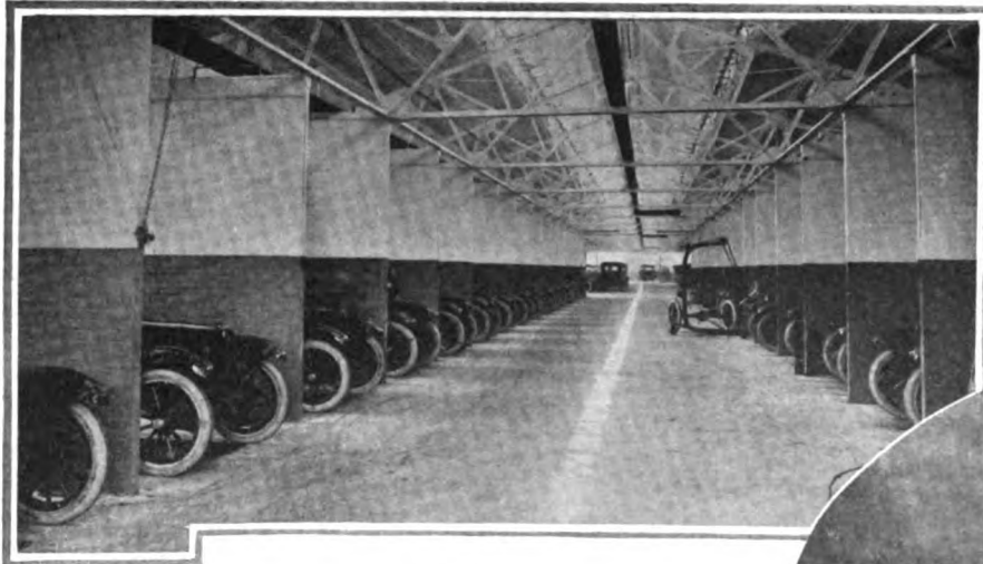
Above is illustrated a testing shed of the Dodge Bros. plant, Detroit, Mich. Solid brick partitions which are practically sound-proof form a series of stalls on each side of the center aisle. After the car has been tested on the track it is run in one of these stalls and the tester is able to detect and remedy the faintest knock
